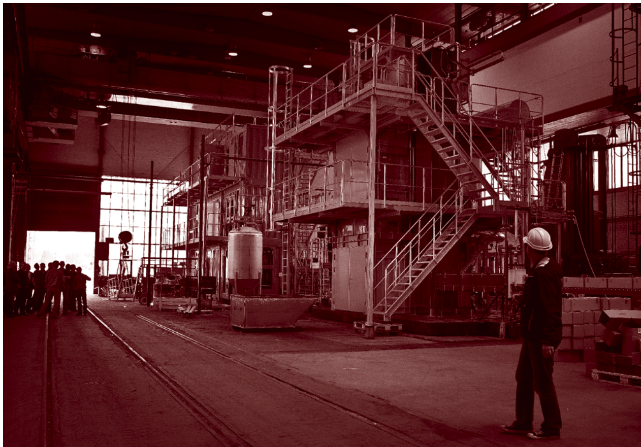
Dynasafe's SDC 1500 for the destruction of conventional ammunition with a capacity of 4.5 kg NEO per feed, Abu Dhabi, 2011. © Dynasafe Demil Systems AB
