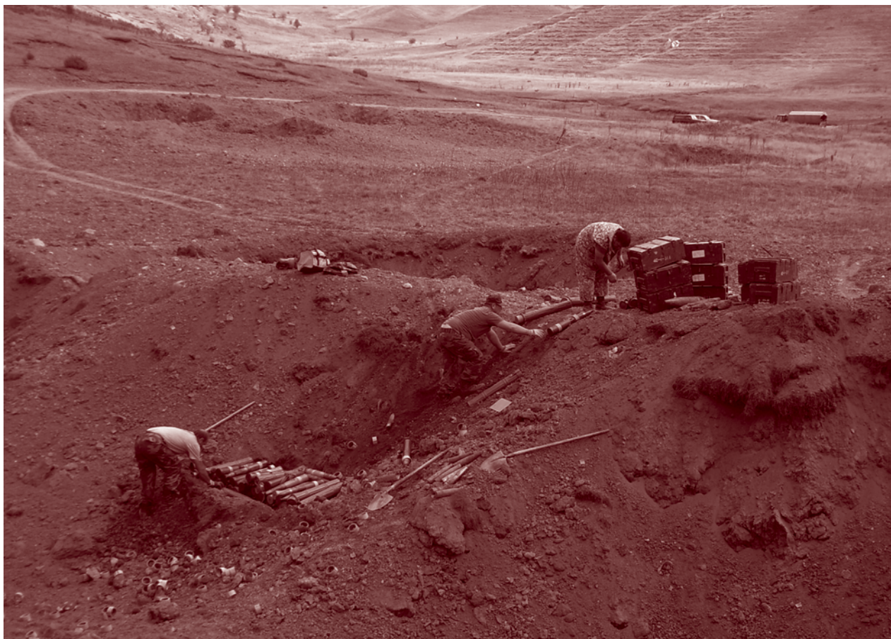
Albanian EOD soldiers preparing a mixed demolition pit of about one tonne of munitions deemed unsuited for industrial demilitarization, Bize demolition range, Albania, September 2009. © David Towndrow, NATO Support Agency (NSPA)
